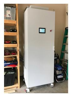
MICROGRID IN A BOX: The Energy Switch combines 5,500 watts of energy storage with circuits that limit the power draw from the grid and also correct for distortion produced by appliances and electronics in the home. The system also manages power from rooftop solar and backup generators when needed.
